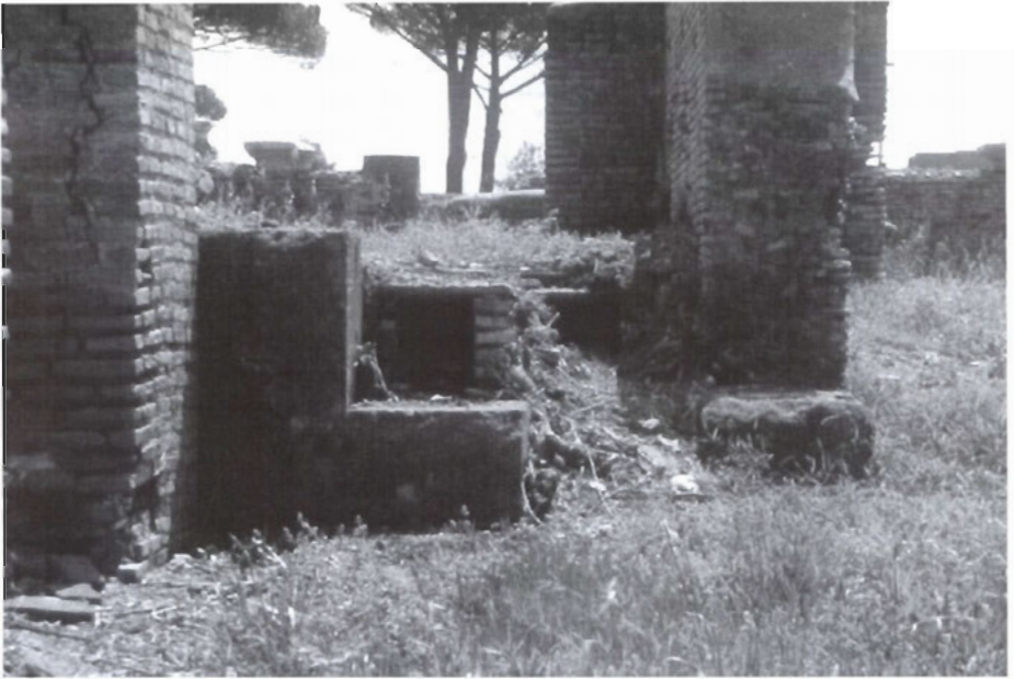
Figure 2. Suspensurae flooring in the Grandi Horrea.
