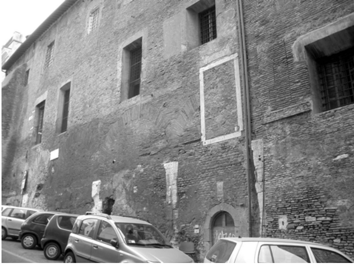
Figure 7: Ancient travertine pillars and brick arches at the Via in Selci (by author).
