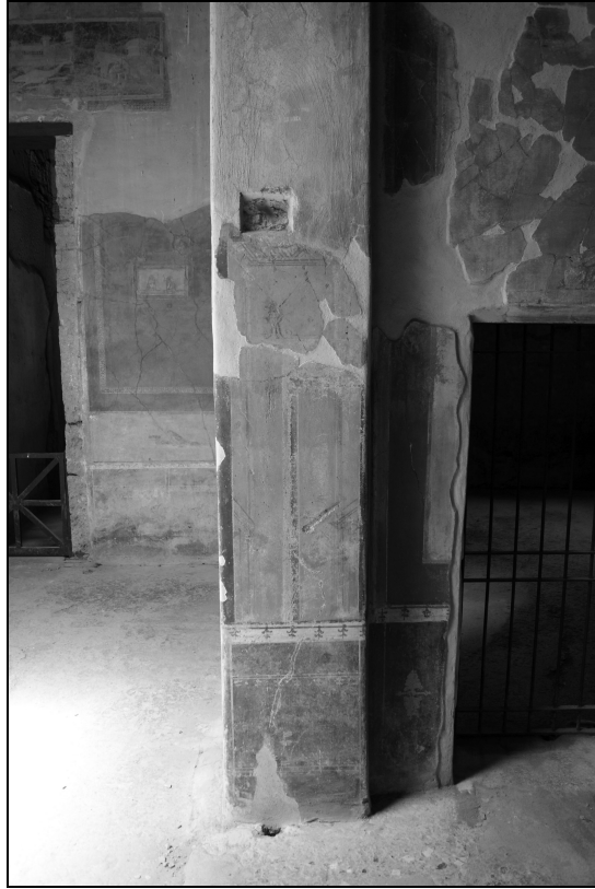
Figure 3: Cuts for a partition in the tablinum, Casa del Menandro (photo by author).
