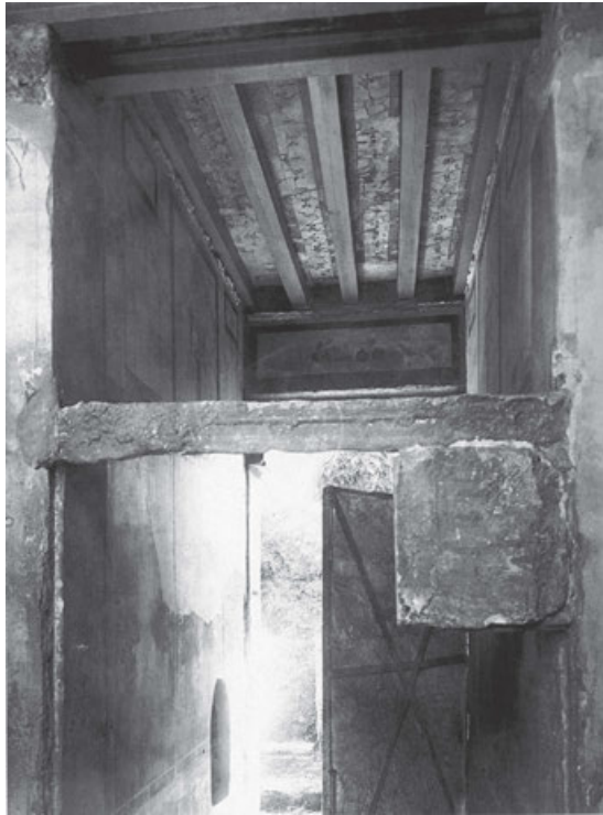
Figure 7: Partial plaster cast of the tri-valve inner entrance door of the Casa dei Ceii (I.6.15). (Archival photograph; SAP photo inv. Pompei B/343). (Reproduced by permission of the Ministero per i Beni e le Attività Culturali. Further reproduction or duplication by any means or methods is prohibited)
