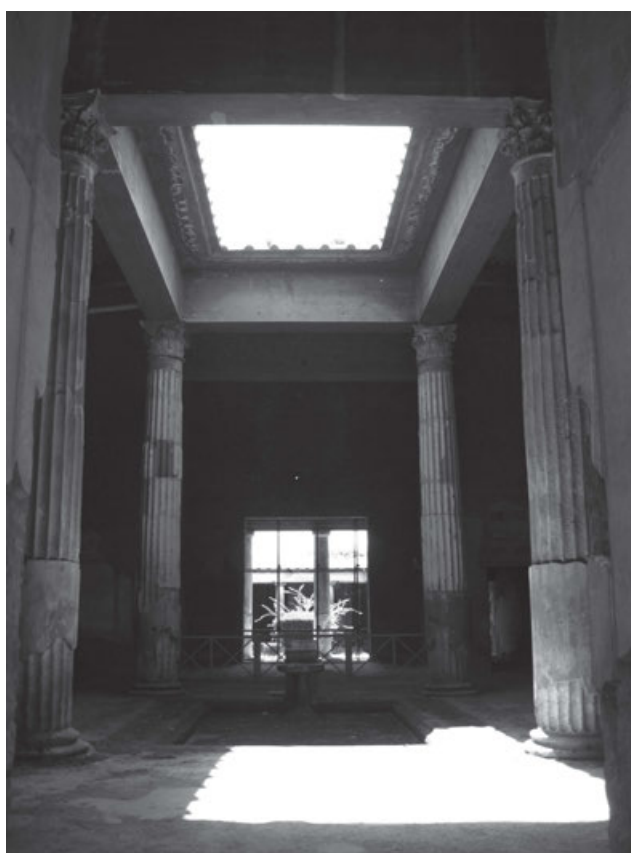
Figure 2: An axial view through the Casa delle Nozze d'Argento (V.2.i) from the main entrance. In its A.D. 79 configuration, the entrance passage was closed by doors at both ends. The front jambs of the tablinum had possible curtain or partition fittings (a pair of figured bronze discs with protruding ship bows (Sogliano 1892: 274; Sogliano 1896: 424; Mau 1893: 33), and the rear of the tablinum was closed by a solid-panel, quadri-valve door (Mau 1893: 33). (Photo by the author)
