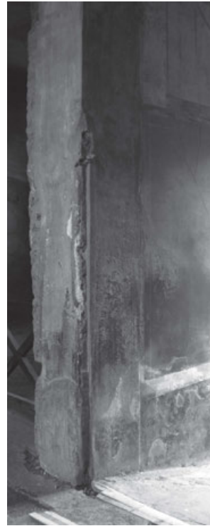
Figure 8: East jamb of the inner entrance doorway of the Casa dei Ceii (I.6.15), showing the approx. 2m tall vertical scar in the plaster on the rear, inner edge of the jamb left by the decayed wooden door frame. (Photo by the author)
