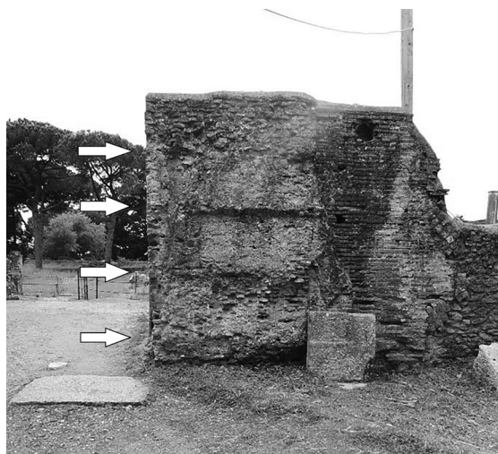
Figure 8: The common wall between the Domus of Apuleius and the theater. The arrows shows the traces of excised blocks (author's photo).
