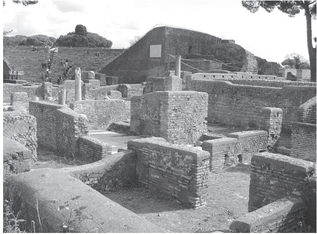
Figure 7: Particular of the domus walls characterized by different kind of masonry (author's photo).
