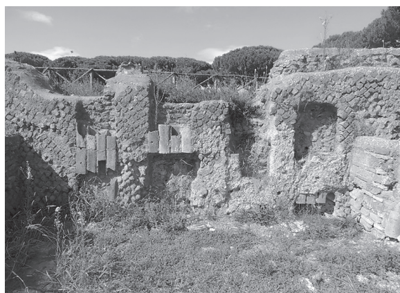
Figure 5: Domus of Apuleius. Particular of the back wall in opus quasi reticulatum altered in a late phase of the domus (author's photo).
