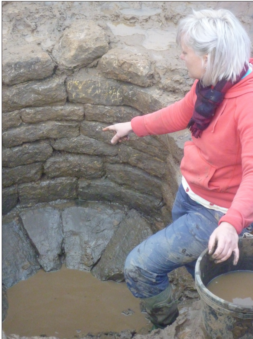
Figure 5: W2 at end of its investigation showing stone base and coursed stone lining (Source: OnSite Archaeology).
