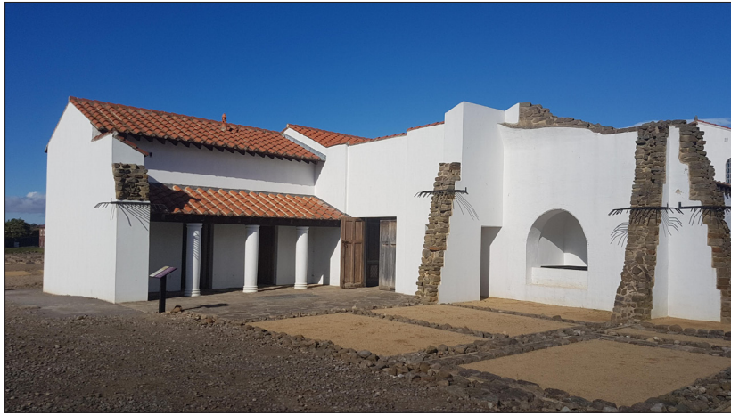
Figure 6: View of the entranceway of the Commanding Officer's House. The area to the right shows the part of the building that was not reconstructed. (Author).
