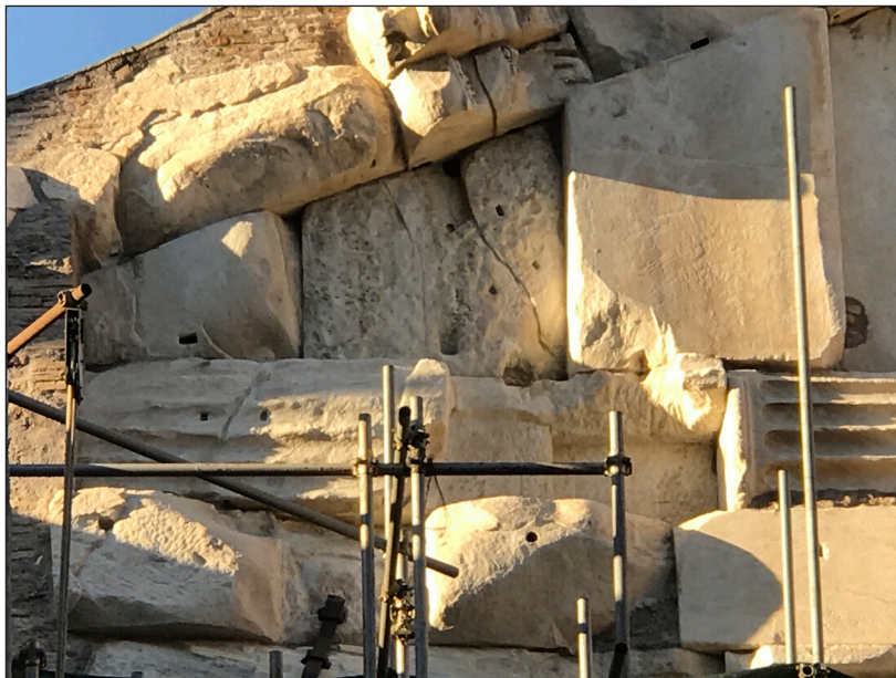
Figure 1: Porticus of Octavia, detail of inner pediment of propylon, showing salvaged column shafts used as building material in AD 203 (Author’s photo, 2017).
