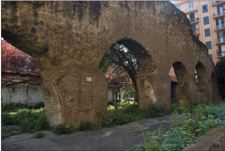
Figure 9: Concrete complex by the Aventine, identified as the Navalia (Author's photo, 2008).
