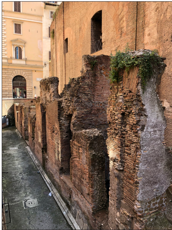
Figure 14: Probable Hadrianic refacing of the Porticus Argonautarum 's rear wall (Author's photo, 2018).
